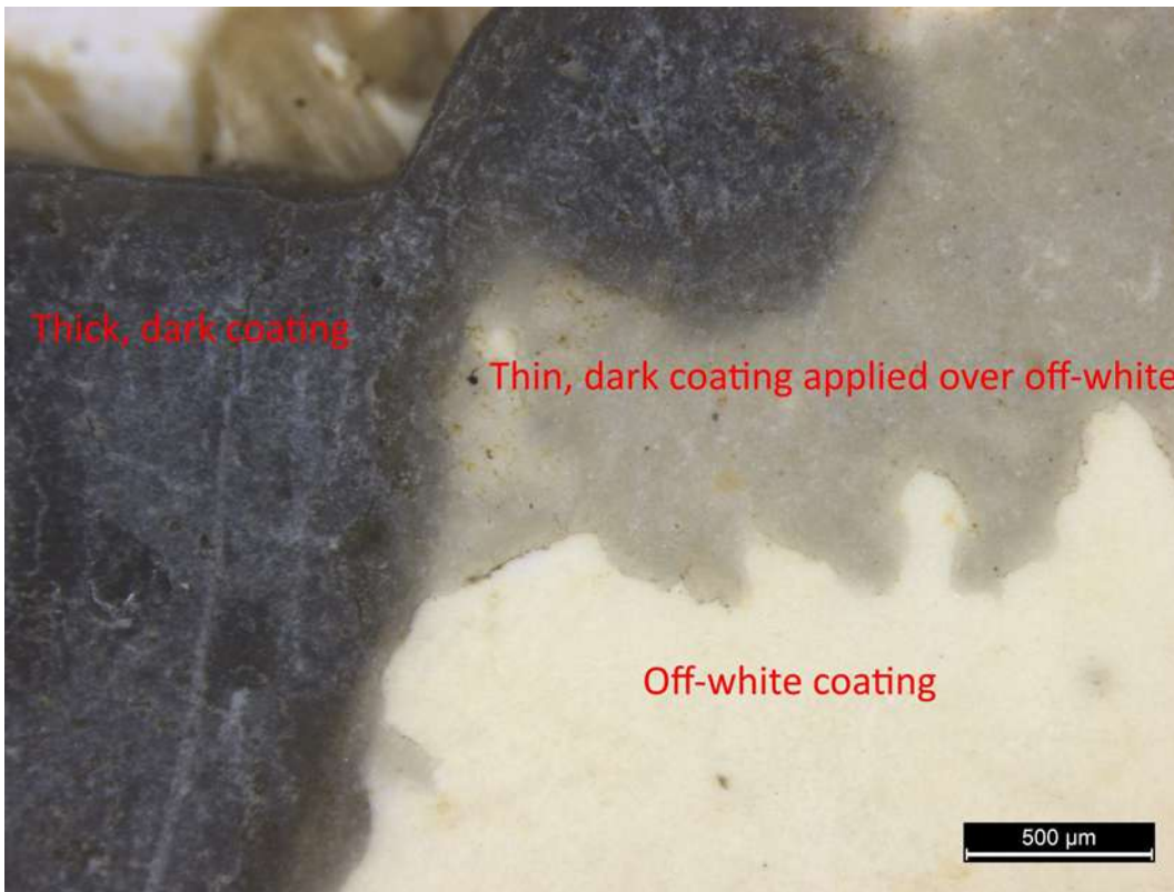
Figure 4: Close-up of applied coatings
